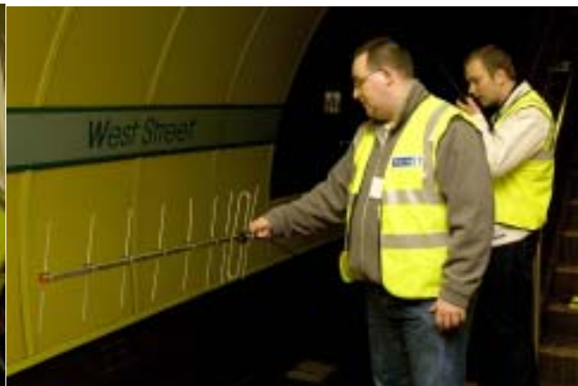
VHF & UHF tests into the tunnels
